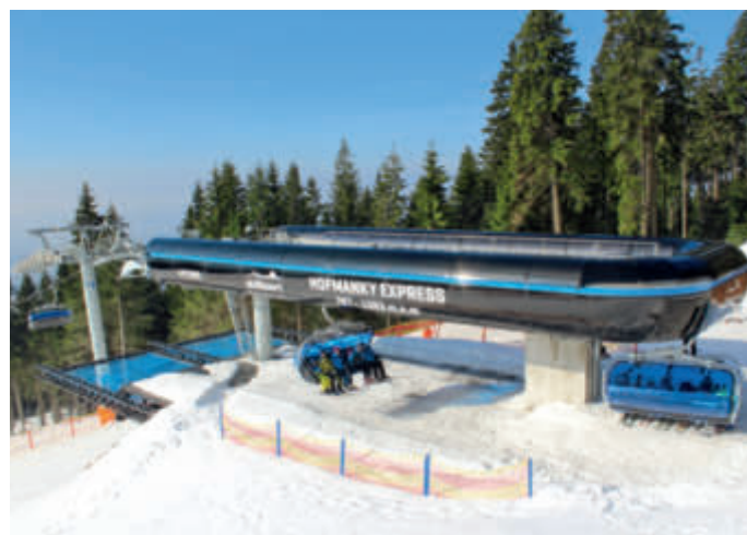
The top station of the Hofmanky Express, which is located on a steep slope, has 90° unloading.
