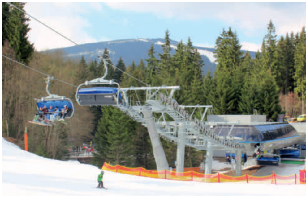
Immediately above the bottom station, a double hold-down tower and a supporting tower provide extra rope height above the piste.
