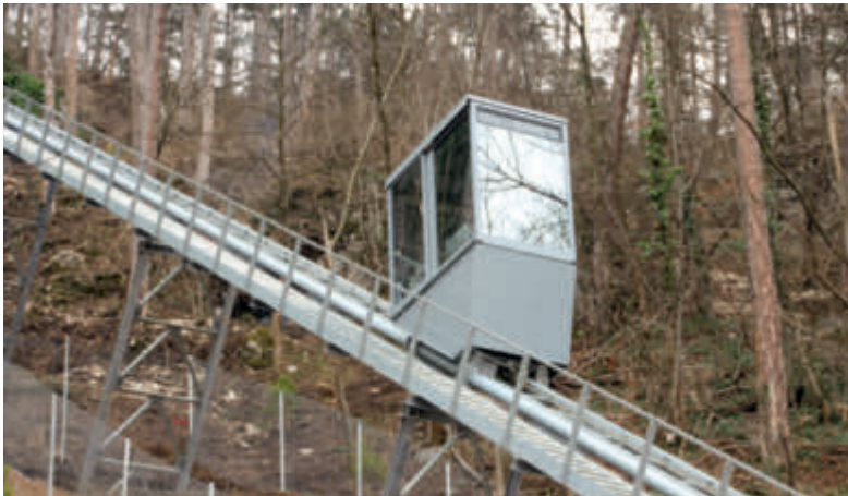
In Râșnov, the inclined elevator from the Comfort series is designed to carry twenty passengers. Since the official opening in June 2015, it has made almost 39,000 trips without a hitch.
