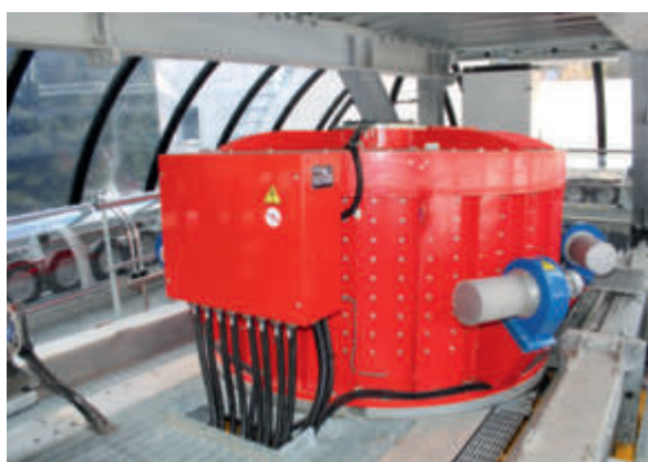
The 668 kW direct drive from Leitner ropeways on the Svatý Petr - Pláň chairlift is currently the most powerful ropeway drive in the Czech Republic.
