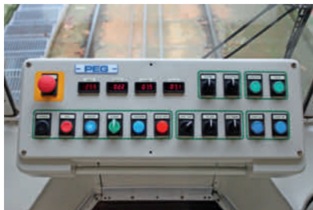
A new control system was installed in 2018.
