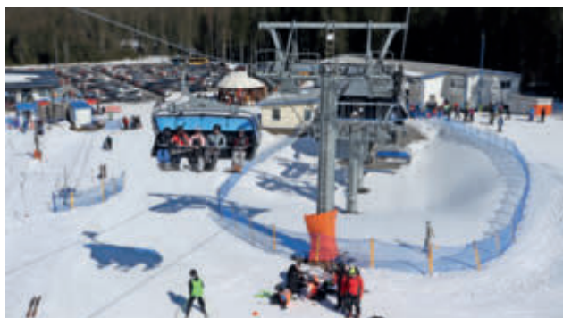
Overall view of the bottom station, with the carrier parking shed and staff rooms in the background on the right
