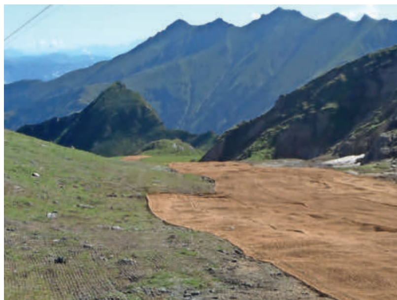
The Aquasol KGW 400 system ensures that the conditions for renaturation and growth are significantly improved and revegetation measures can be successful.
