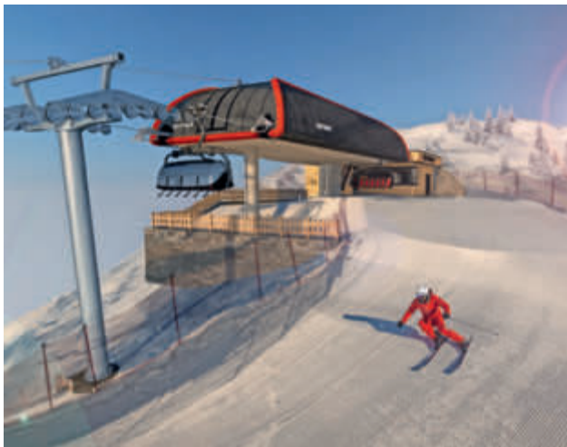
Top station of the new Gauxjoch lift. The 6-seater chairlift is due to open in December 2023.
