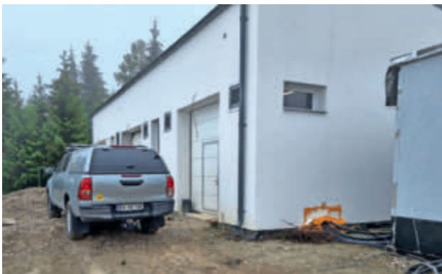
The main pump station under construction just below the storage pond
