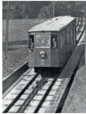
In 1932 the funicular was rebuilt and the line extended to its current length.
