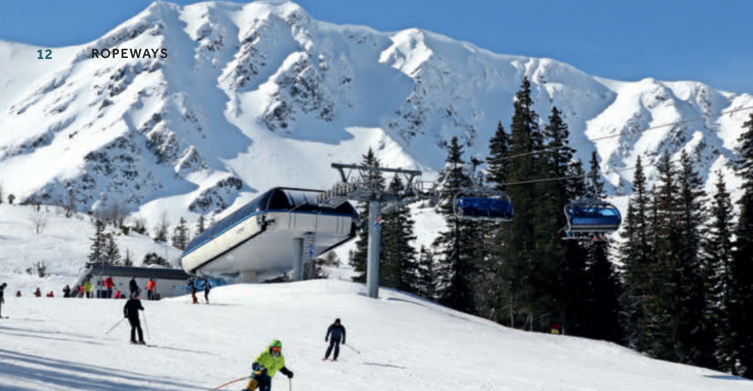
Top station of the Roháče Express 6-seater chairlift with Salatín (2,048 m) providing an impressive backdrop
