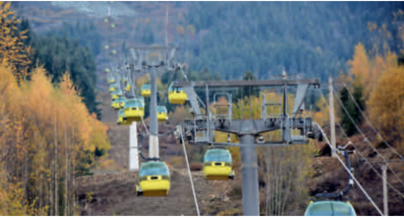
The finished 8-seater gondola lift prior to issue of the operating permit
