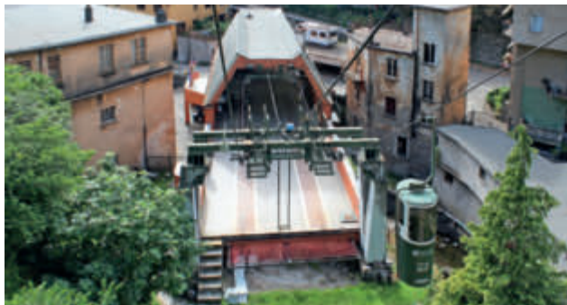
The bottom station is located in the middle of the built-up area of Laveno
