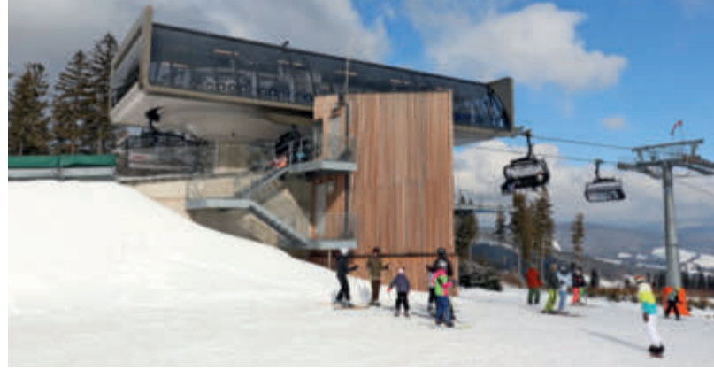
... and top station of the Stříbrnice-Štvanice 6-seater D-Line chairlift
