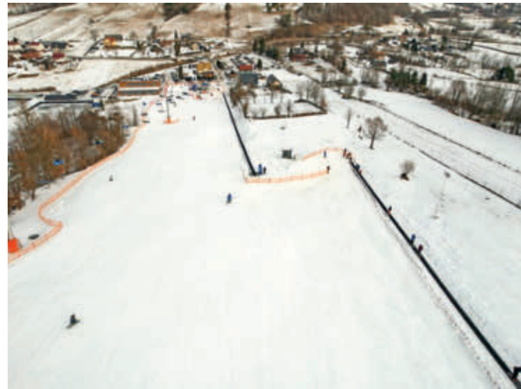
Moving carpet no. 1 serves as a feeder to moving carpet no. 2 at Bieszczad Ski. The two moving carpets of the same length offer easy access for beginners to the slope along the line of the chairlift.
