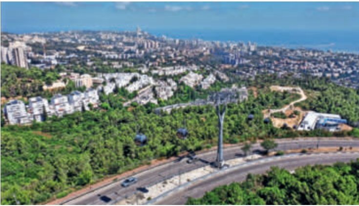
Passengers ride the almost 4.5 km long line up to Mount Carmel in just 19 minutes – with no traffic jams and a fabulous view of the sea.
