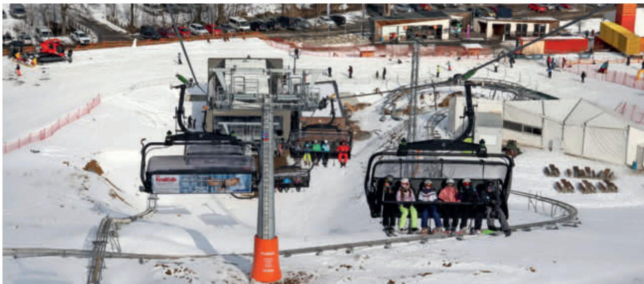
The first D-Line chairlift in the Czech Republic is now operating in the Kraličák ski area (here looking towards the bottom station).
