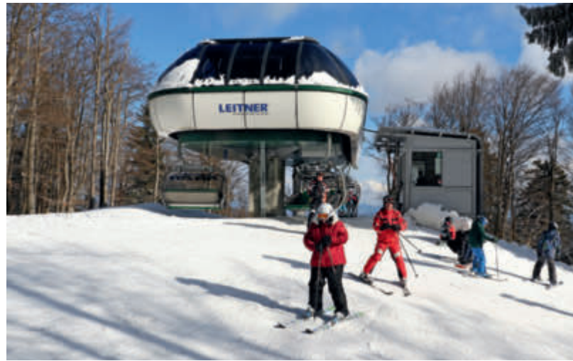
The top station of the Buková hora chairlift is a return station with a high enclosure.
