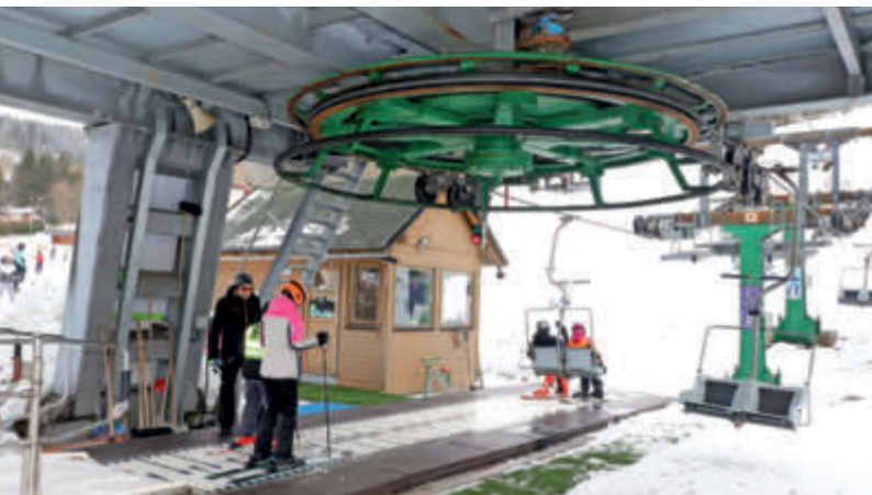
The used double chairlift on the Čenkovice side was fully refurbished prior to installation in the area.
