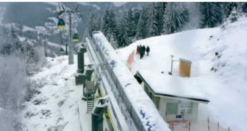
View from a cabin on the downhill line of the mid station located on the uphill line
