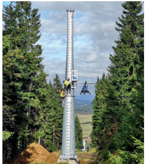
A helicopter was used to install the towers in difficult terrain.
