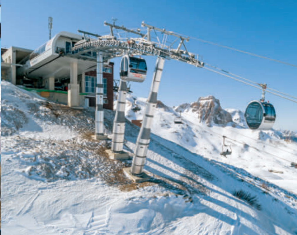
Equipped with 96 gondolas, the new BergJet can carry around 2,200 passengers per hour to the Maschgenkamm. It offers convenient and barrier-free all-year access to the mountain peak for a variety of excursions.
