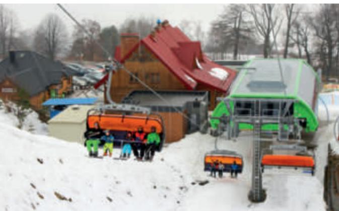
Bottom station of the Kasina Wielka 6-seater chairlift
