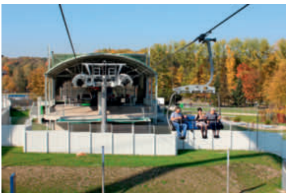
The basement drive is located in the Silesian Stadium Station and the carrier parking shed behind it.
