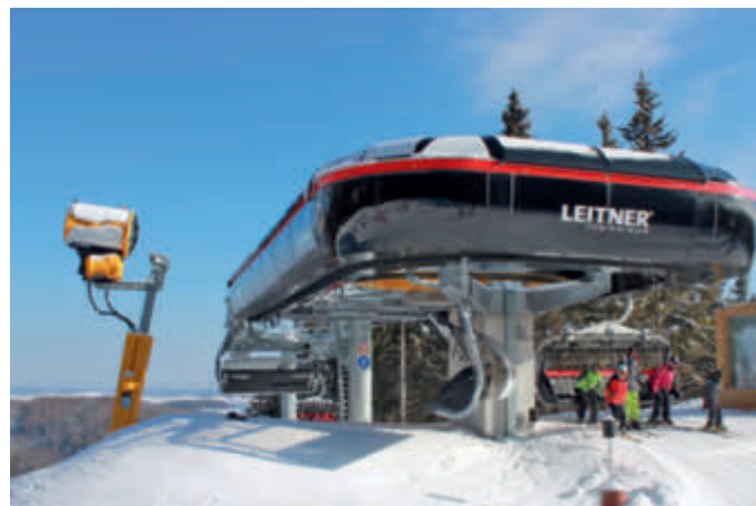
Top station with the compact enclosure is located at 881 m a.s.l.; on the left one of the new TF10 snow guns from Technoalpin
