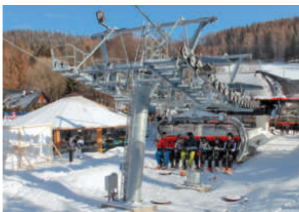
Bottom station with the two compression towers
