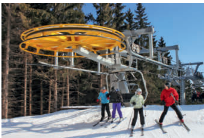
Top station of the fixed-grip quad chairlift built in 2012, which will reopen in the Mosty u Jablunkova Ski Area in the winter of 2018/19
