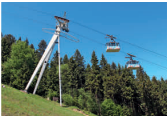
The cabins at the mid-point of the line, with the unusual steel-plate tower on the left
