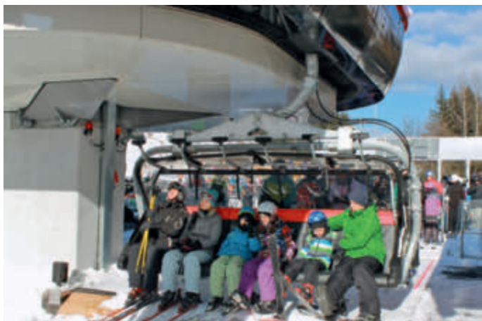
90° loading in the bottom station with the height-adjustable loading carpet that matches the children's height to the approaching chair
