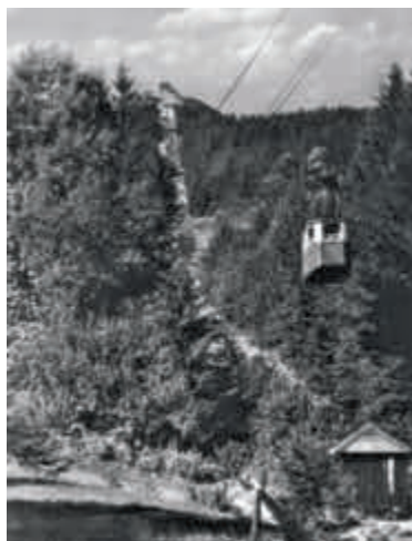
View of the complete line of the old reversible from the bottom station
