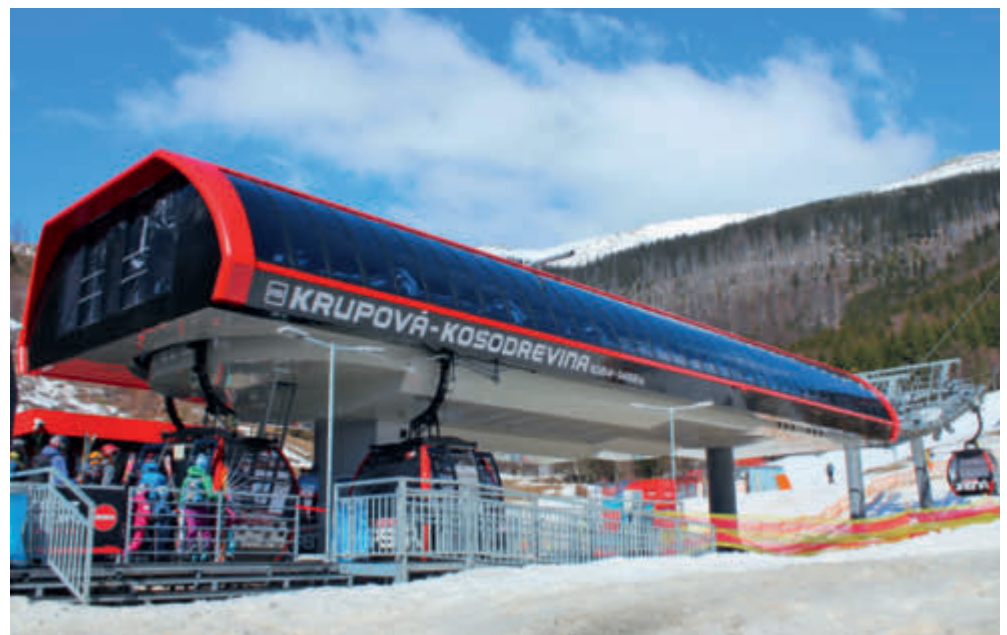
The open bottom terminal is a UNI-G design located at 1,089 m a.s.l.
