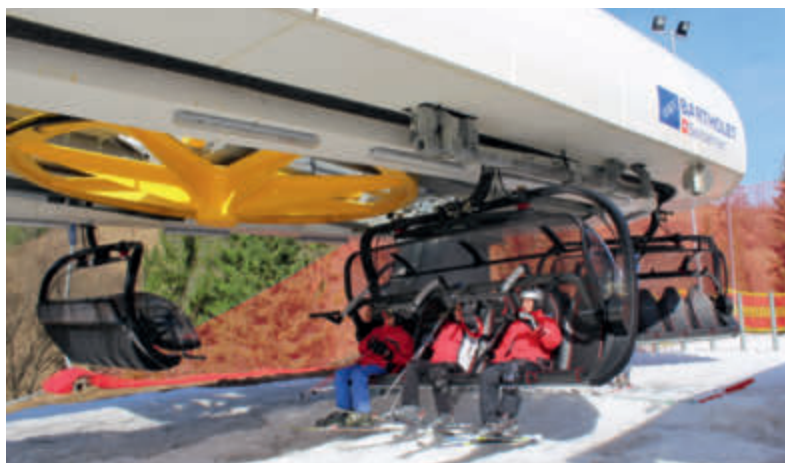
The bottom station of the Bartholet 6-seater chairlift at Rusin-ski is a deflection station with a low enclosure.
