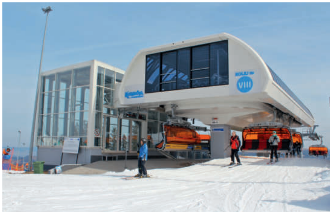
Basement parking (left) for all 53 chairs on the Jankulakowski 6-seater chairlift in Białka Tatrzańska
