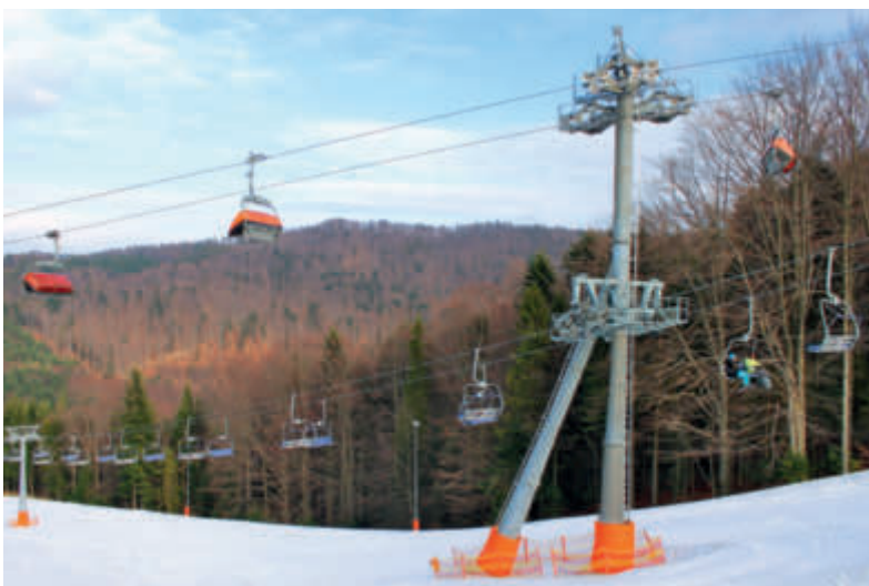
The intersection of the Czarny Groń 1 fixed-grip quad chairlift and the Czarny Groń Express detachable 6-seater chairlift on a shared tower.
