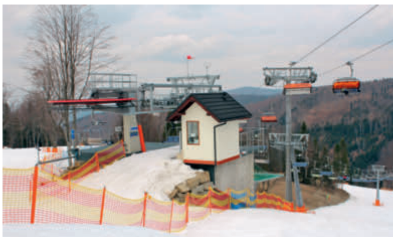
In the Czarny Groń Ski Area, the fixed-grip four-seater chairlift and the detachable 6-seater chairlift with protective canopies intersect on a shared tower near the upper terminal of the quad.
