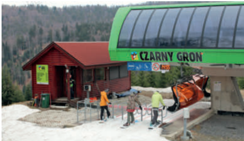
90° loading carpet solution for the Doppelmayr 6-seater chairlift at Czarny Groń
