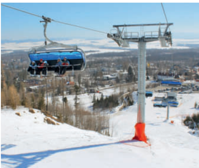
The Tatranská Lomnica – Buková Hora 8-seater chairlift with padded seats, the Kidstop seat guard for children and blue canopies, on the Slovak side of the High Tatras
