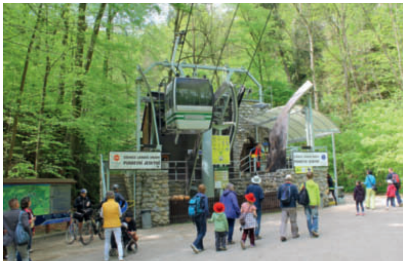
From the bottom station near the old car park, the line rises at a gradient of up to 100 percent.
