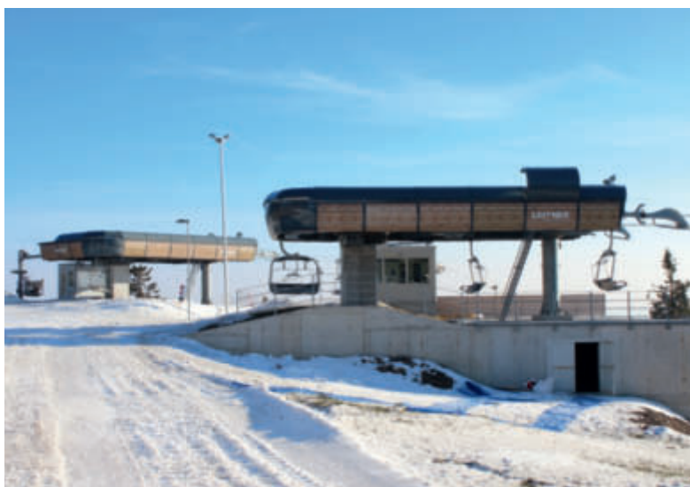
Leitner Ropeways supplied no fewer than three new quad chairlifts to the new Plešivec Ski Area in the Ore Mountains (CZ). The photo shows the upper terminal of the two detachable installations, with the longest – the Pstruží – Plešivec chairlift – in the background and the Modesgrund – Plešivec chairlift in the foreground.
