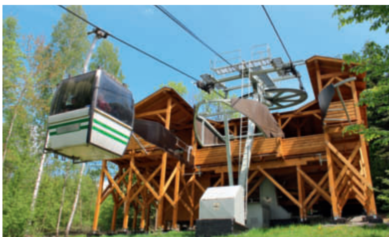
At the beginning of 2015, the old open wooden platform used for the upper station was replaced by a wooden building.
