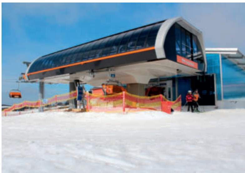
Upper terminal of the new Jáchymov – Klínovec quad chairlift (for marketing purposes also called the Prima Express), with automatic carrier parking
