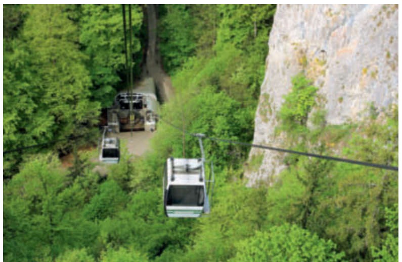
View from the tower of the steep line up the sheer face of the gorge
