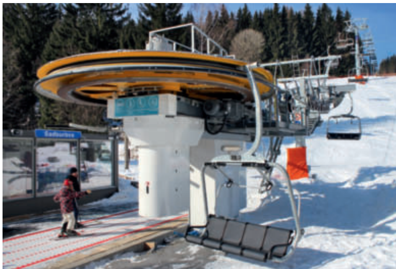
The Kopřivná fixed-grip quad chairlift – in the photo the lower terminal with Unifix drive – serves the Kopřivná family trail in Malá Morávka.
