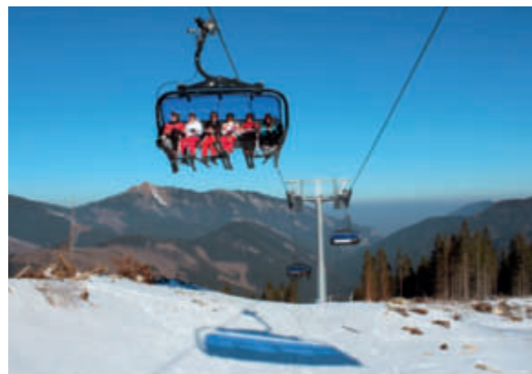
The new Leitner 6-seater chairlift serves as an access system from the car parks in Lúčky and as a repeat-ride installation for the family trail.
