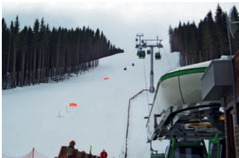
View from the bottom station along the line of the first stage of the gondola ropeway
