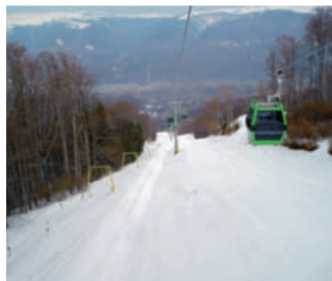
In 2012 a new gondola for easier access to the Straja ski area was built as a public investment.
