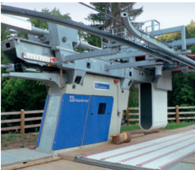
The bottom station of Ruia Chairlift, loading with conveyor belt
