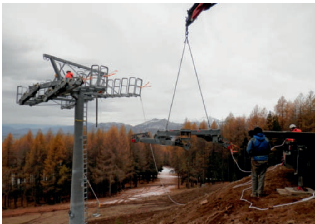
LST chairlift at Rosa Khutor resort under construction
