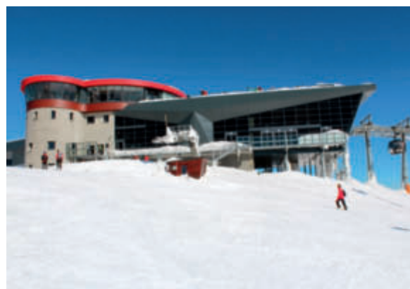
The upper terminal of the 15-seater gondola ropeway from Kosodrevina to Chopok (built in 2012) was integrated in the new mountain lodge.
