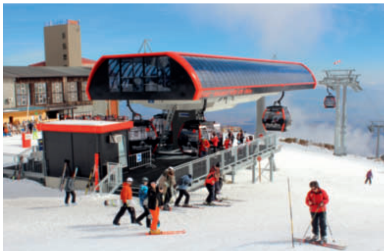
The upper terminal of the 15-seater gondola ropeway to Skalnaté Pleso was built next to the old station with direct access to the ski trails. The old terminal building has been converted into an events location, an information center and gallery, and a viewing tower.
