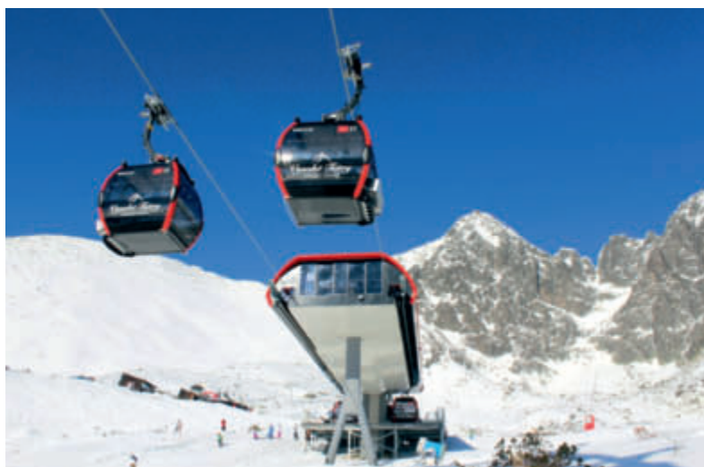
Upper terminal of the new Doppelmayr 15-seater gondola ropeway from Štart to Skalnaté Pleso, with Lomnický Peak (2,634 m) in the background
