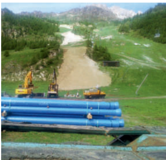
The Val d'Isère snowmaking system upgrade using Duktus pipes
