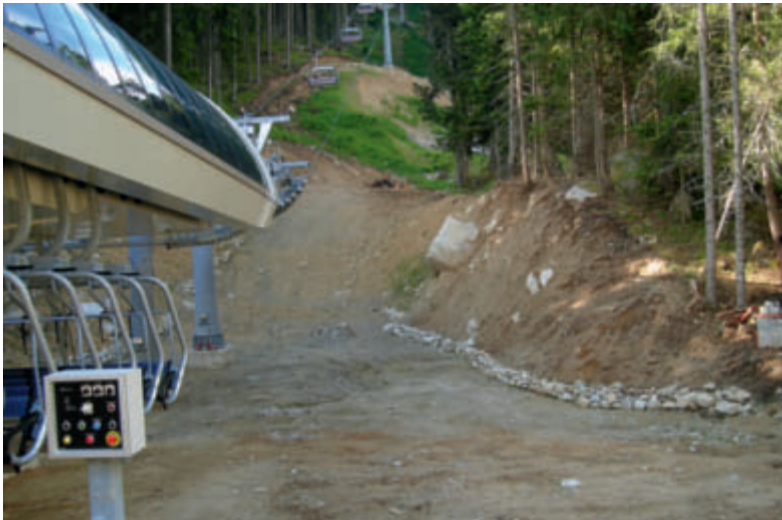
The slope near the lower terminal in spring 2011 ...
