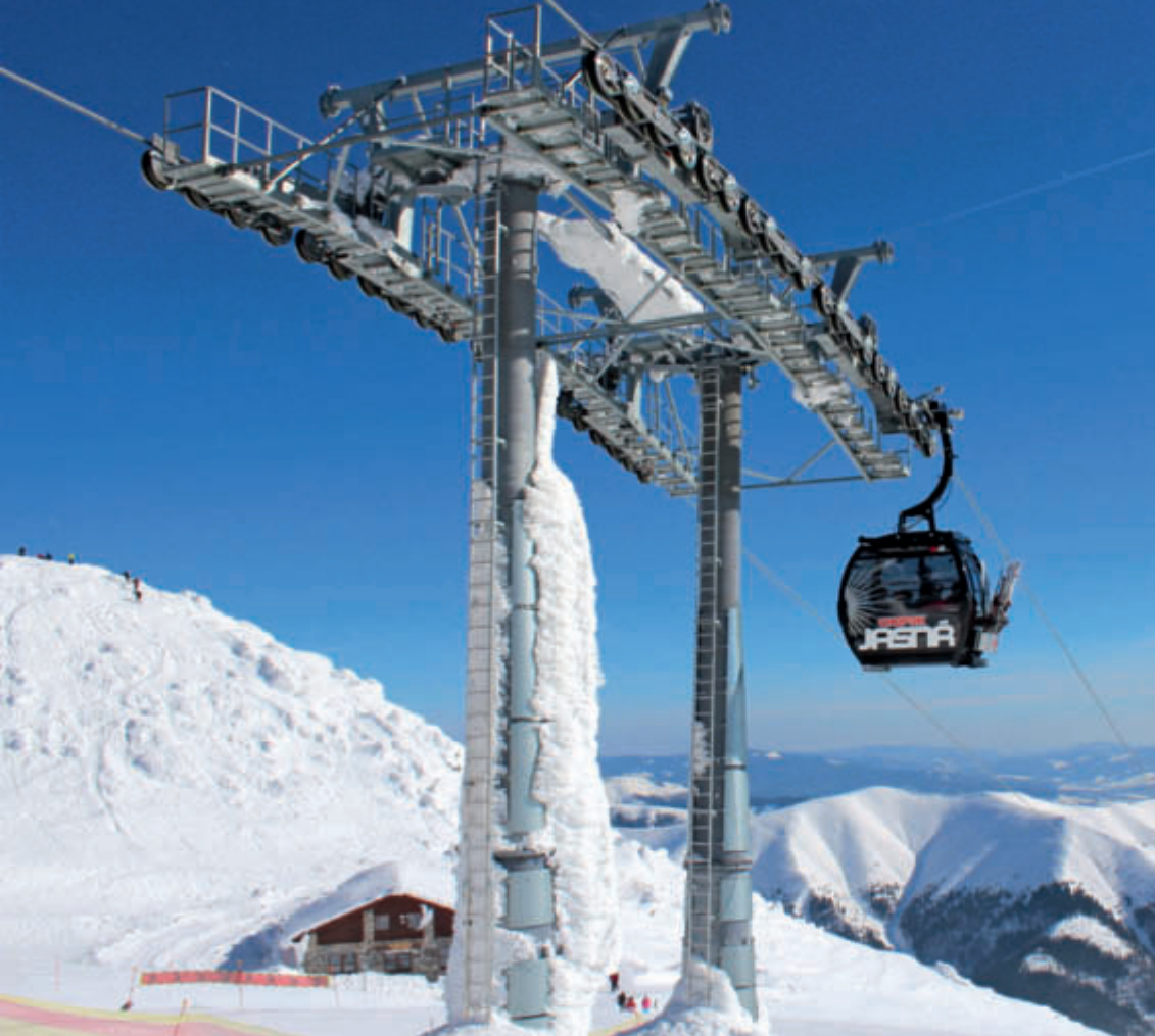
The new 15-passenger cabins on the Kosodrevina – Chopok ropeway near the upper terminal
