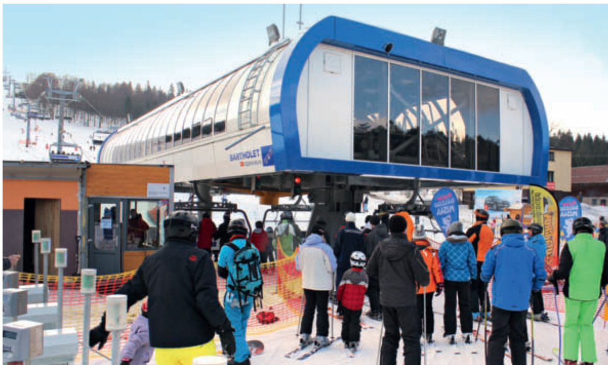
Lower terminal of the Złoty Groń 6-seater chairlift with the drive and hydraulic tensioning system
