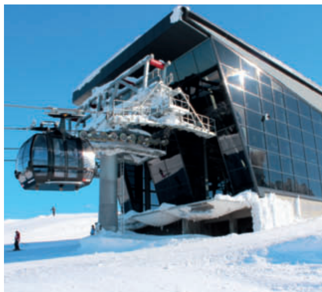
The fully galvanized structure of the upper terminal of the Funitel on Chopok with its dark glazing matches the black design of the cabins.
