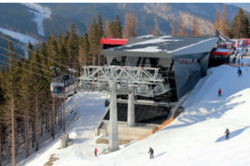
Particular importance was attached to the architecture of the lower terminal. Between the terminal and the first tower, visitors can observe the underground drive through the glazed roof. The red roof to the left belongs to the upper terminal of the Twinliner.
